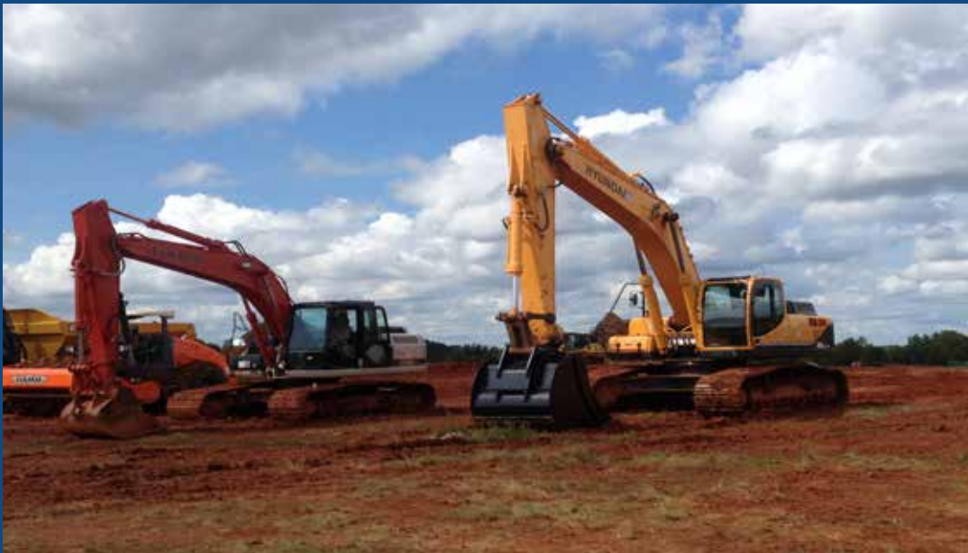
New construction equipment on site of future hospital.
